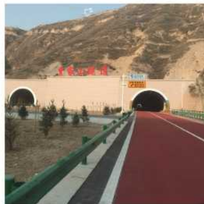
Lanzhou Highway Tunnel, China
