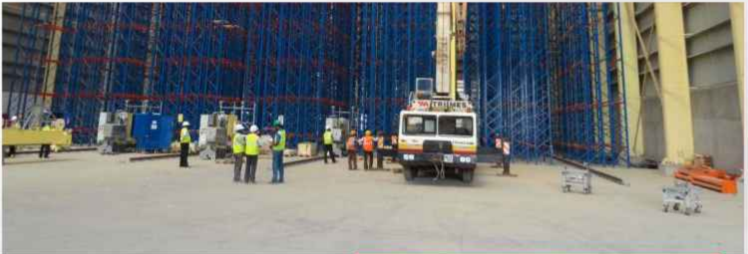
Super Flat Floor for 30m High Racking with ASRS
