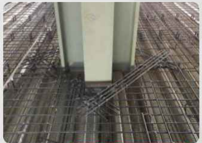
Detailed Engineering for Deck Slab Flooring
