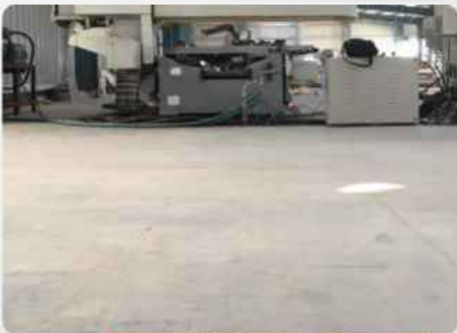
Deck Slab for Manufacturing Industry
